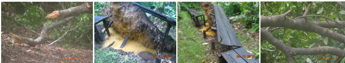
Fig. 17, 18, 19& 20 show cross section of the trees that fell across the boardwalk
