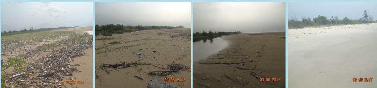
Fig 17, 18, 19&20 shows impact of coastal erosion and encroachment at the shoreline
