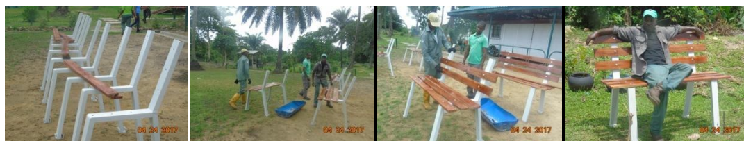
Fig.16, 17, 18 & 19 show pictures of the Rangers during the seat-out construction work
