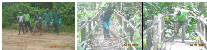
Fig. 13, 14, & 15 show cross section of the Rangers during the boardwalk trimming and cleaning exercise
