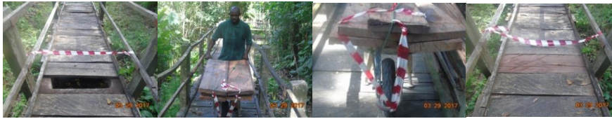
Fig. 13, 14, 15 & 16 shows Cross section of the damaged trails and repair
