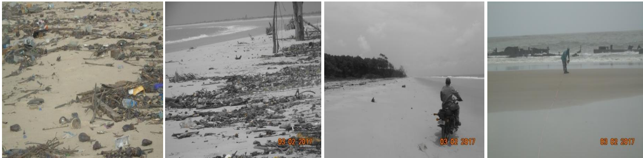
Fig 17, 18, 19&20 shows photos of impact of coastal erosion and encroachment at the shoreline and Park rangers during monitoring of Coastal erosion
